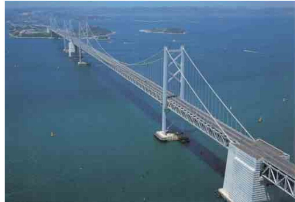
Seto Ohashi Bridge
