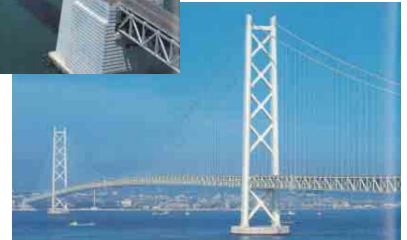
Akashi Kaikyo Ohashi Bridge
