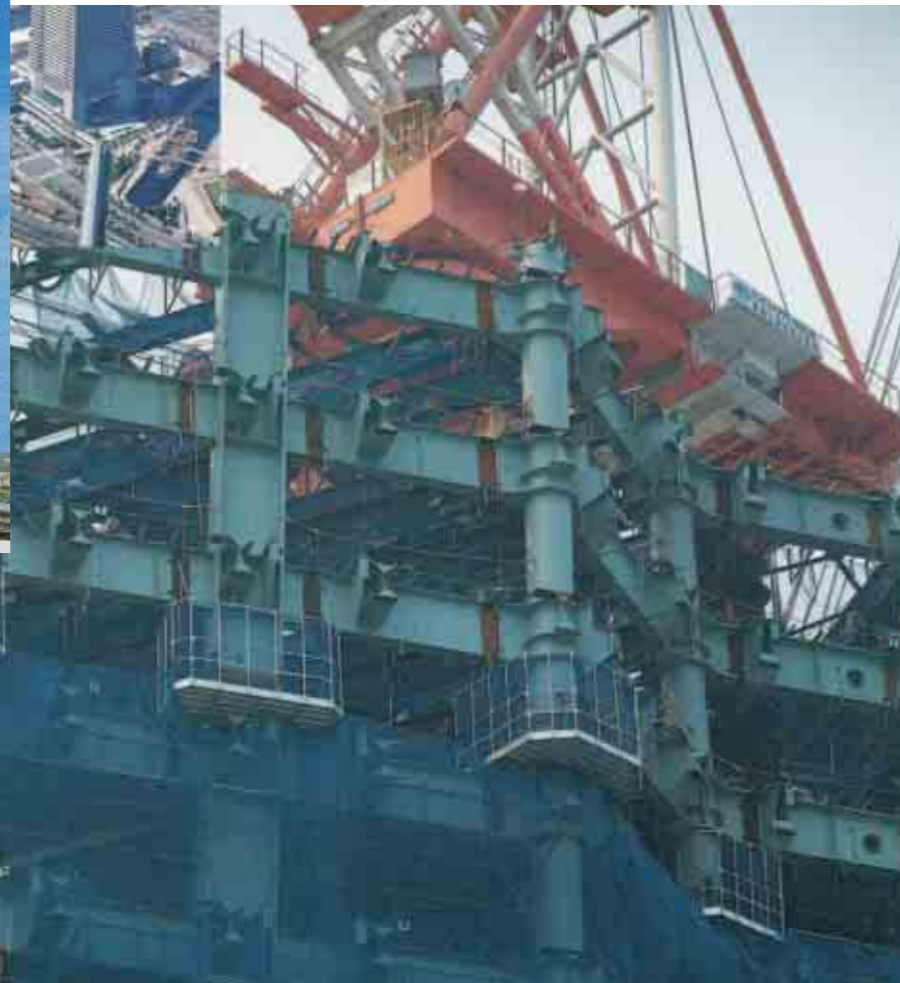
Steel frame construction in Yokohama Landmark Tower
